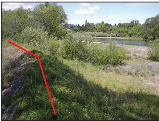
Figure 10. Vegetated berm used to prevent facility inundation when the river is at flood stage.
